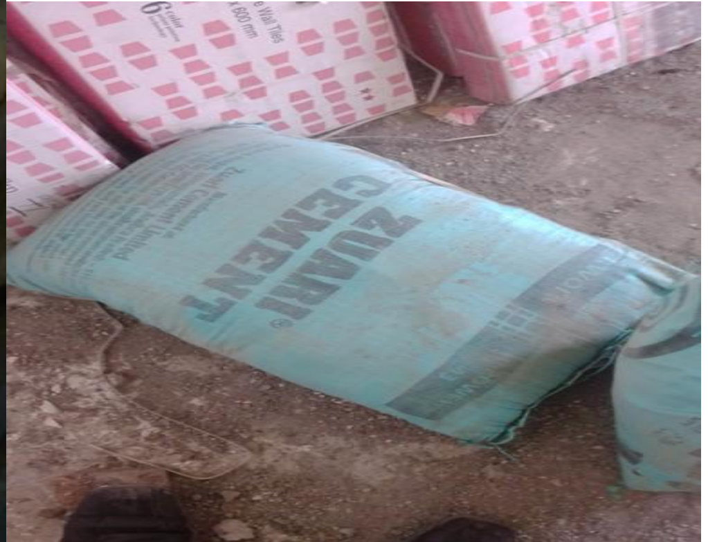
2) Checking the Cement—43-Grade or PPC
