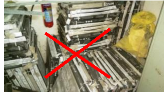
Irregular Stacking may cause the damages
