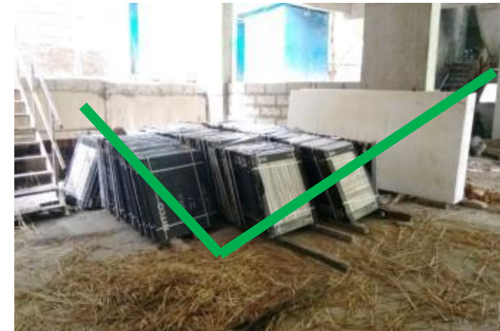
Laying is Perfect in all regards.
