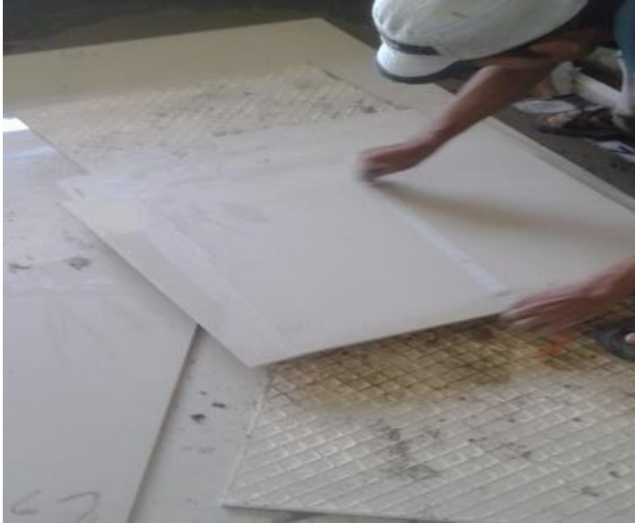
9) Marking for cutting tiles
