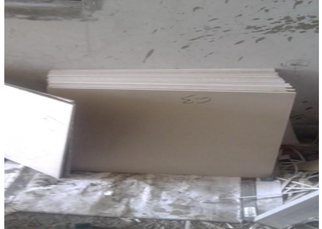
2) Take out the tiles from the boxes
