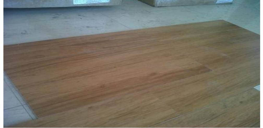
Straight Course Laying No problem
