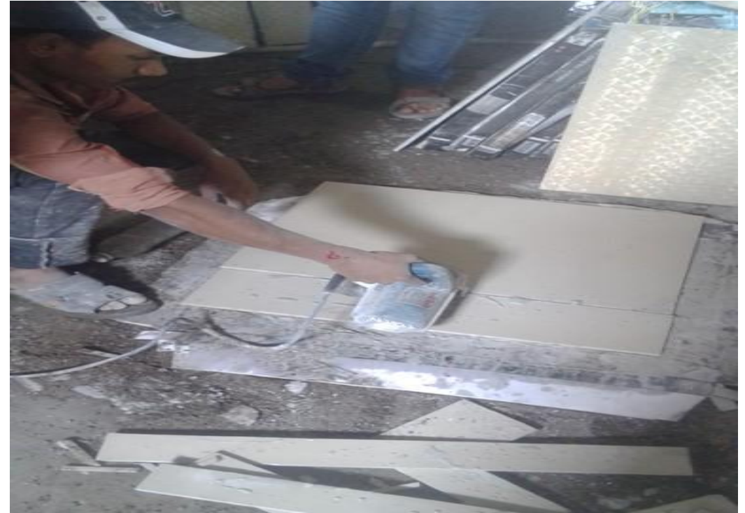
10) Cutt the tiles by Diamond Blade only
