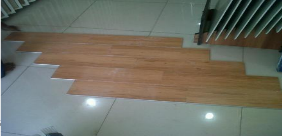
Step Laying &5:25 off set Right pattern
