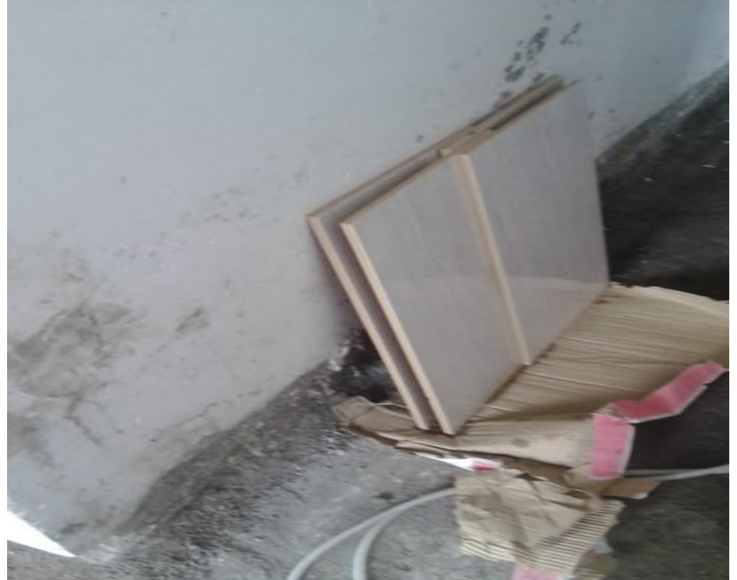
4) Dry the tiles after soaking.
